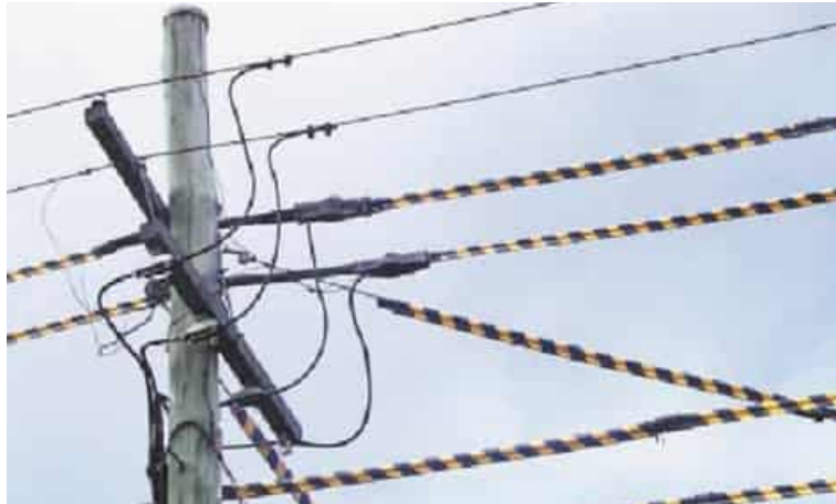
Figure 16 – Tiger tails fitted to overhead power lines
