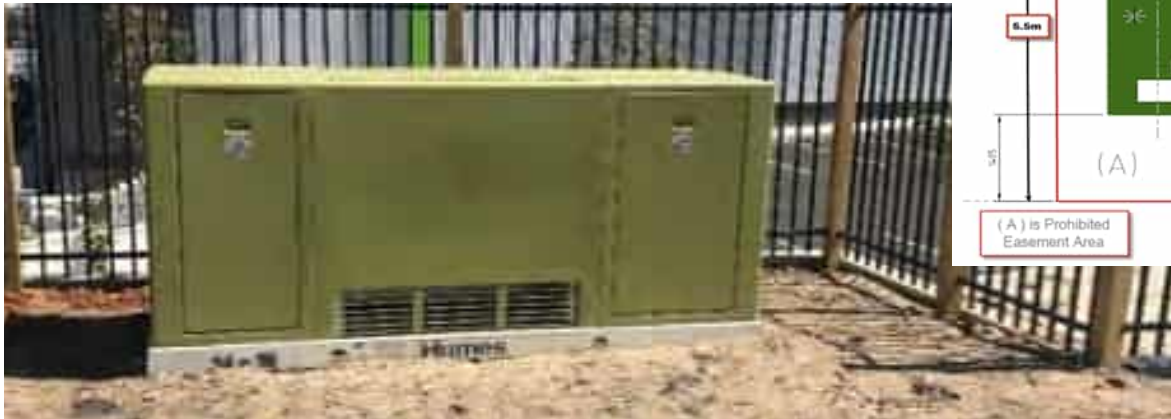
Example of a padmount substation
