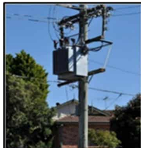
Pole mounted substation
