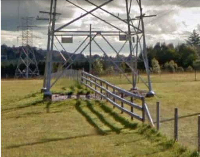
Poor subdivision of easements restricts access and working area around the structures. Source: Google Maps Street View.
