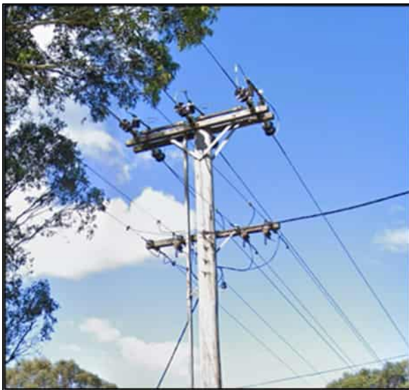
High and low voltage overhead mains
