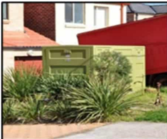
Padmount substation
