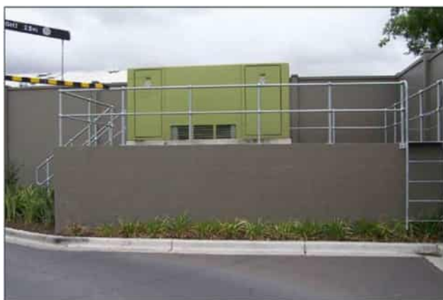
Figure 51 - Example substation raised above 1:100 flood level
